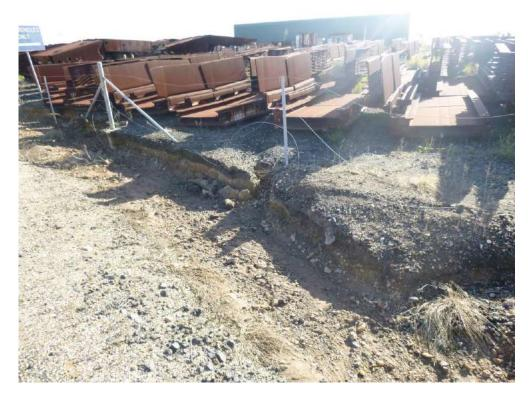
Photo 15 Some minor erosion repairs required around the Pit Top
