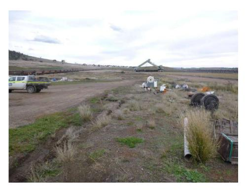
Photo 7 Minor shaping of drainage line required to direct water to sediment dam.
