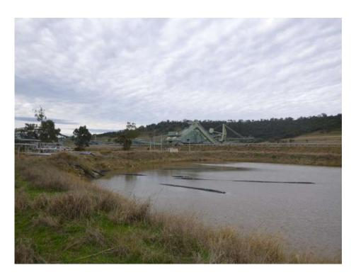
Photo 8 Eastern Dam is the main sediment storage at CHPP
